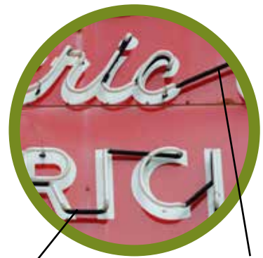
Block-out paint should be applied to define letter forms and tube ends. Eventually this paint will peel off and should be reapplied.
